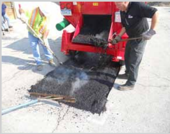
COAT ASPHALT WITH REJUVENATOR
