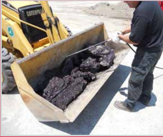
COAT ASPHALT WITH REJUVENATOR
