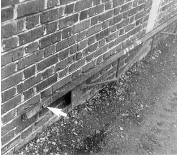
Figure 39: End of a lattice purlin with a bolt hole through the chord.
