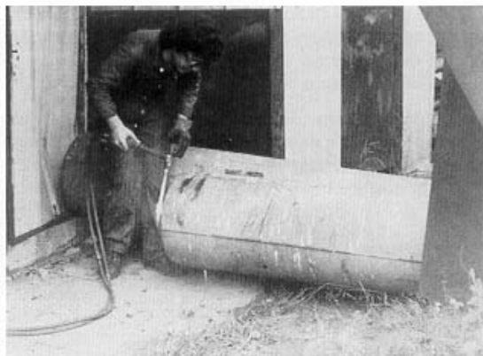
Figure 51: Hall I: single tube semi-portal. Cutting out of the sample
