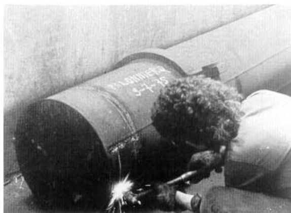
Figure 45: Lifting beam 2 – cutting out of sample
